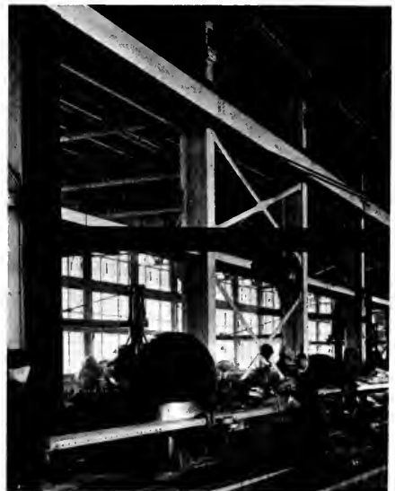
Fig. 8. A 3-ton electric hoist mounted on a jib crane of 35-foot effective reach. The machine is a motor operated friction saw, shown coming into a heavy section 15-inch ship channel. The saw cut through the channel in 15 seconds.
